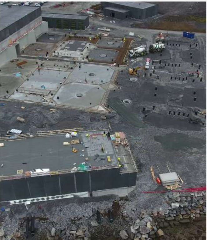
Figure 8.2.2.1 The construction site of Kilvika in 2024. The new smolt facility will be finished and ready for complete use by the end of 2025.
